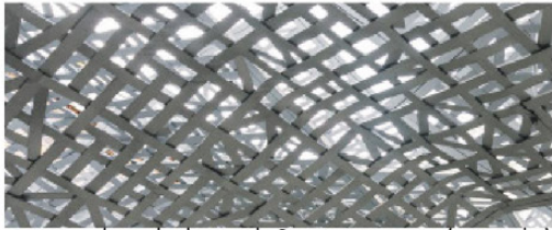
braided metal. Sun protection (pergola)
